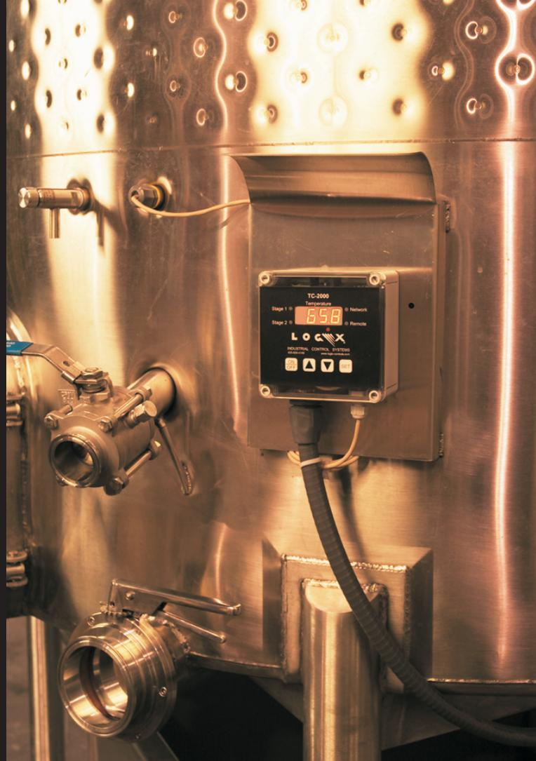
*"The Logix TC-2000 is an ideal winemaking tool. It automates the regulation of your tank temperatures and provides peace of mind through temperature alarming. By adding the computer interface with report-generating capability, you will find it much easier to analyze and repeat your successes."*
